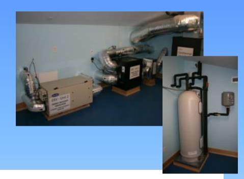
Ventilation Energy Recovery wheel extracts energy from the exhaust air. Dedicated ventilation system allows A/C units to turn off when not needed.
